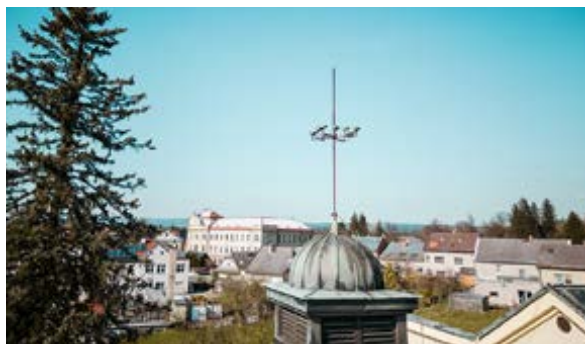
To commemorate the pioneer, a replica of the construction was installed on the roof of a theatre in the Czech town Žamberk that can still be visited today.
