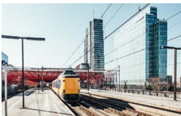
Railway station Almere Centrum
